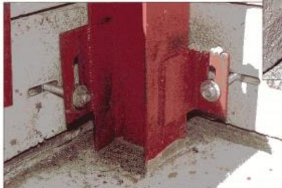
4-WAY ADJUSTMENT BOLTED TO FRAMEWORK.
