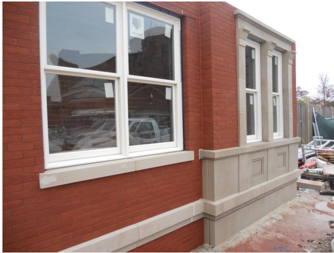
Figure XX. Exterior Mock-Up courtesy of Clark Construction
