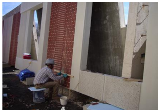
Figure 1.2. Precast plant quality control. Courtesy of PCI
