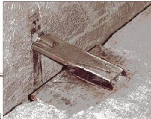
2-WAY ADJUSTMENT WELDED TO FRAMEWORK.
